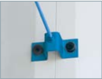
3. Internal reinforcement (Upper piece-PE Sheathed STS)
