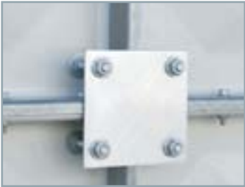
11. External reinforcement (Lower piece-HDG)
