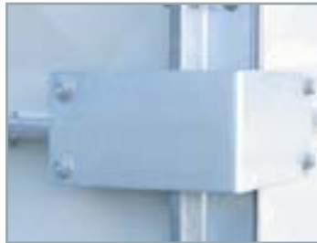
10. External reinforcement (Corner piece-HDG)
