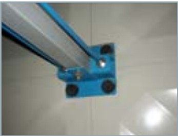
4. Internal reinforcement (GRP rectangular pipe)
