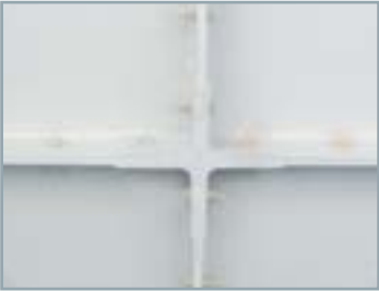
2. Bolts for roof panel (High tensile plastic / Stainless steel)
