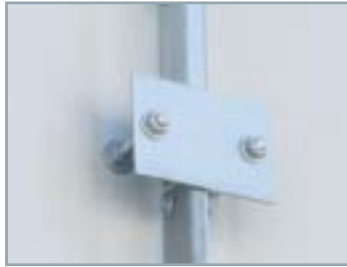
9. External reinforcement (Upper piece-HDG)
